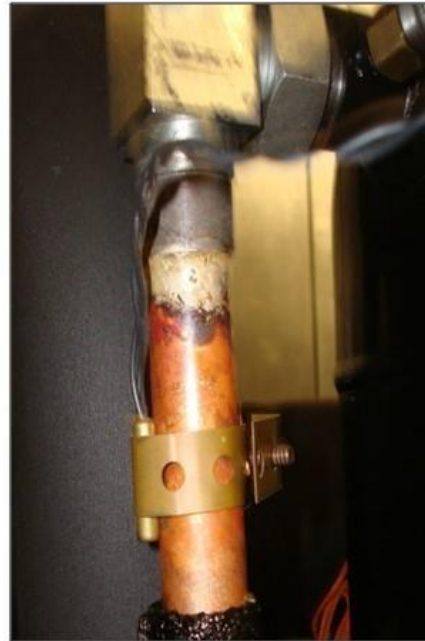
Figure 31 Discharge Line Thermistor
