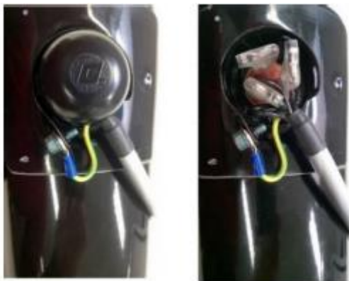
Figure 11 - Terminal dome cover and correct installation, European Electrical
